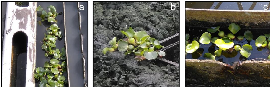
Fig. 3. Eichhornia crassipes placed in a) Primary clarifier, b) Trickle filter, c) Secondary clarifier [24]
